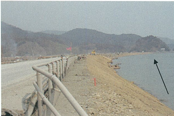
護岸の仮復旧
