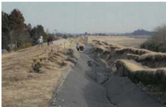
▲鳴瀬川左岸の被災
